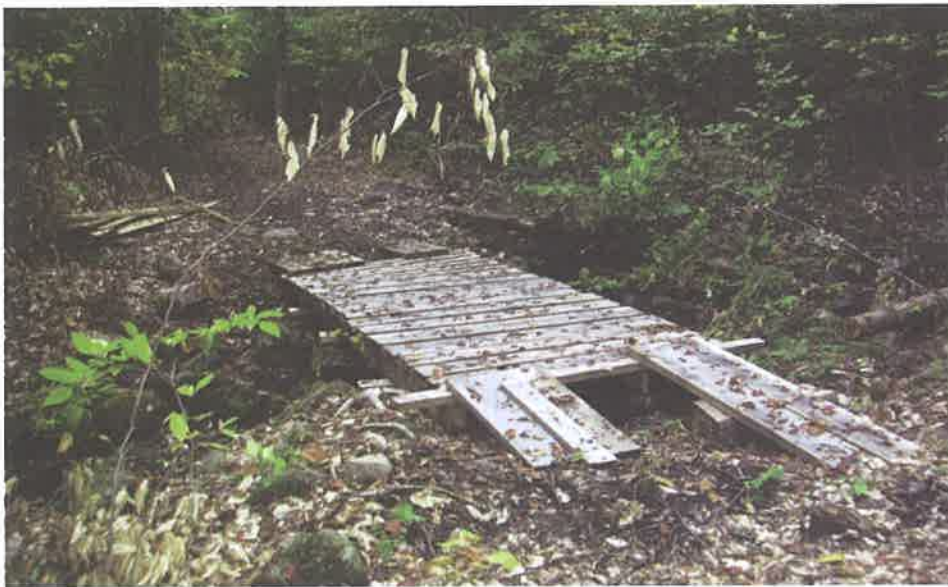
Larry Phillips built this bridge to access additional areas of his property with the tractor without disturbing natural water flows on the land.
